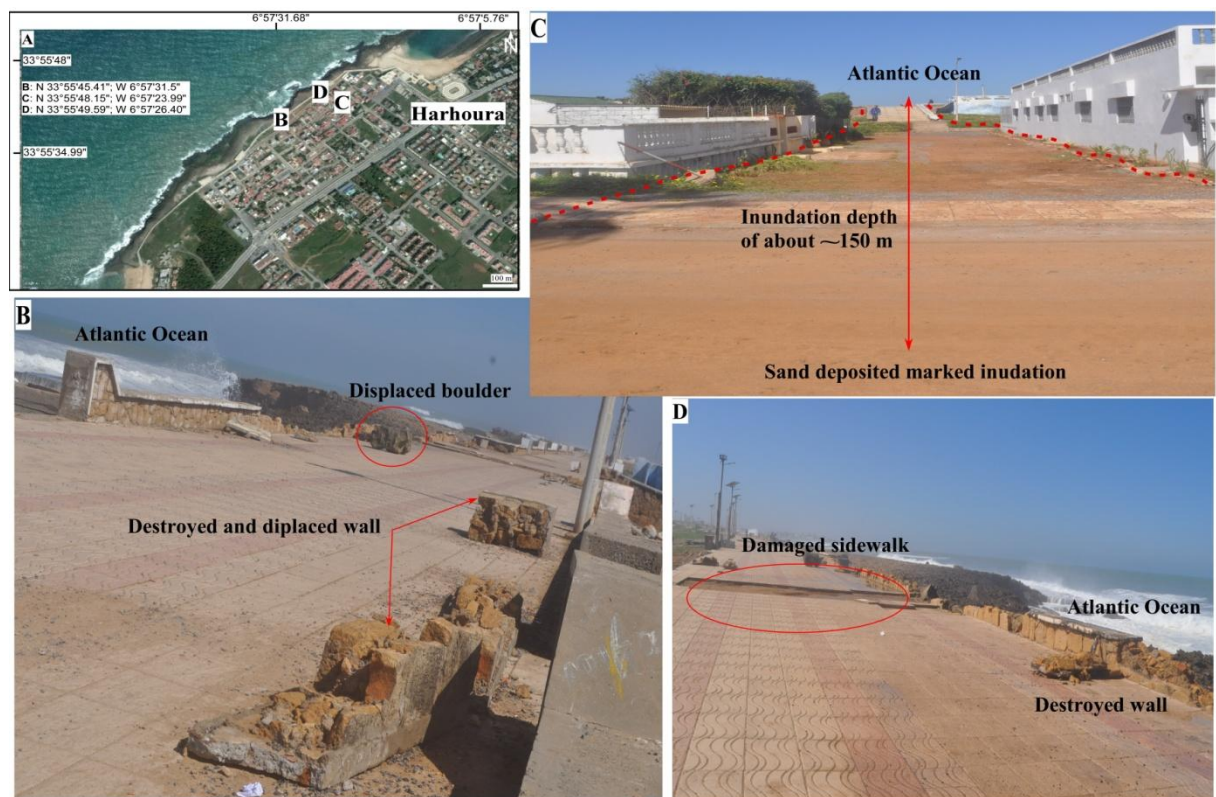
Figure 4. Damage caused by the storm surge on Temara. A: Location of the observation sites; B: Destroyed and displaced wall, displaced boulder (1.4 x 0.8 x 0.5 m); C: inundation marked by sand deposited (~150m); D: Sidewalk and wall destroyed.
